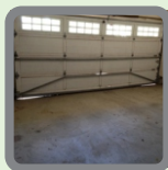
Garage Door Openings
